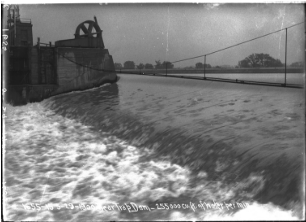
With the Chicago River reversed, a flow of 4,250 cubic feet per second flows over the submerged Bear Trap Dam at Lockport in May 1900. The completion of the decade-long project to construct the Main Channel provided water treatment by dilution for nearly 1.3 million Chicagoans. (Photo courtesy of Metropolitan Water Reclamation District of Greater Chicago)
